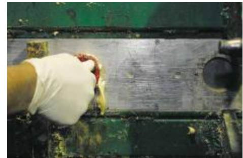
KERI RASMUSSEN / DAILY COMMERCIAL Alex Shaw plugs a wall panel after the polyurethane foam injection process at Insulated Component Structures in Eustis on Wednesday. The foam will expand to fill the panel restricting air movement within the wall. Finished panels are set in a channel that is secured to the foundation and locked together using a cam-lock system.
